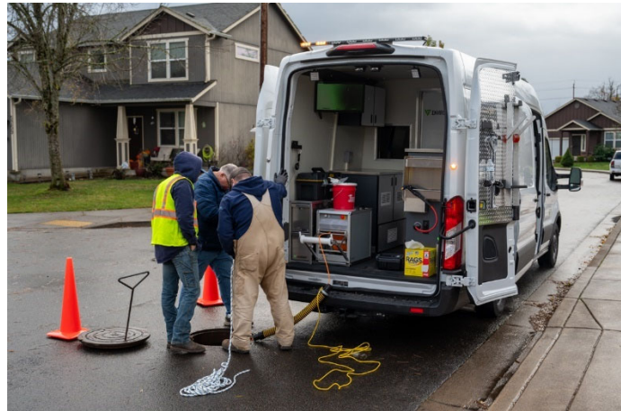
Inspecting wastewater pipe to help prevent costly failures
