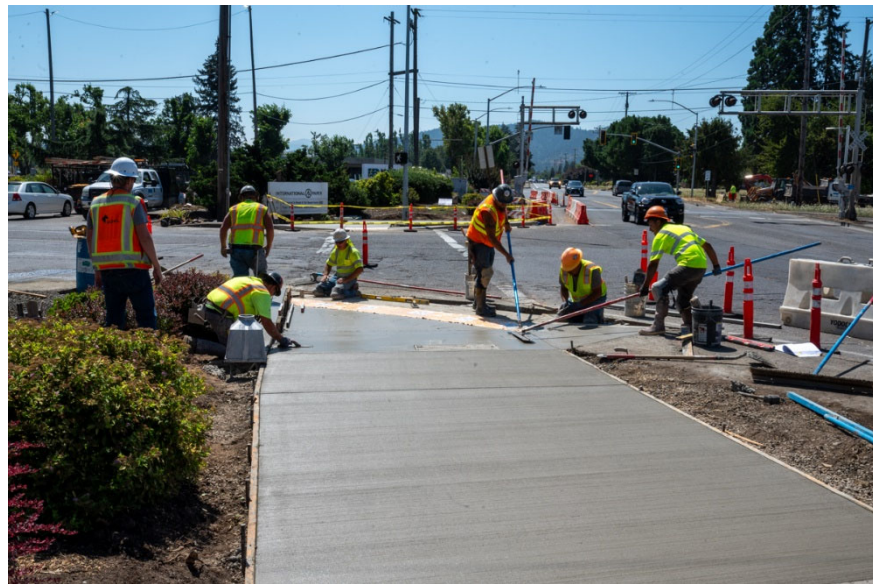
S. 42nd Overlay ADA Ramp Construction
