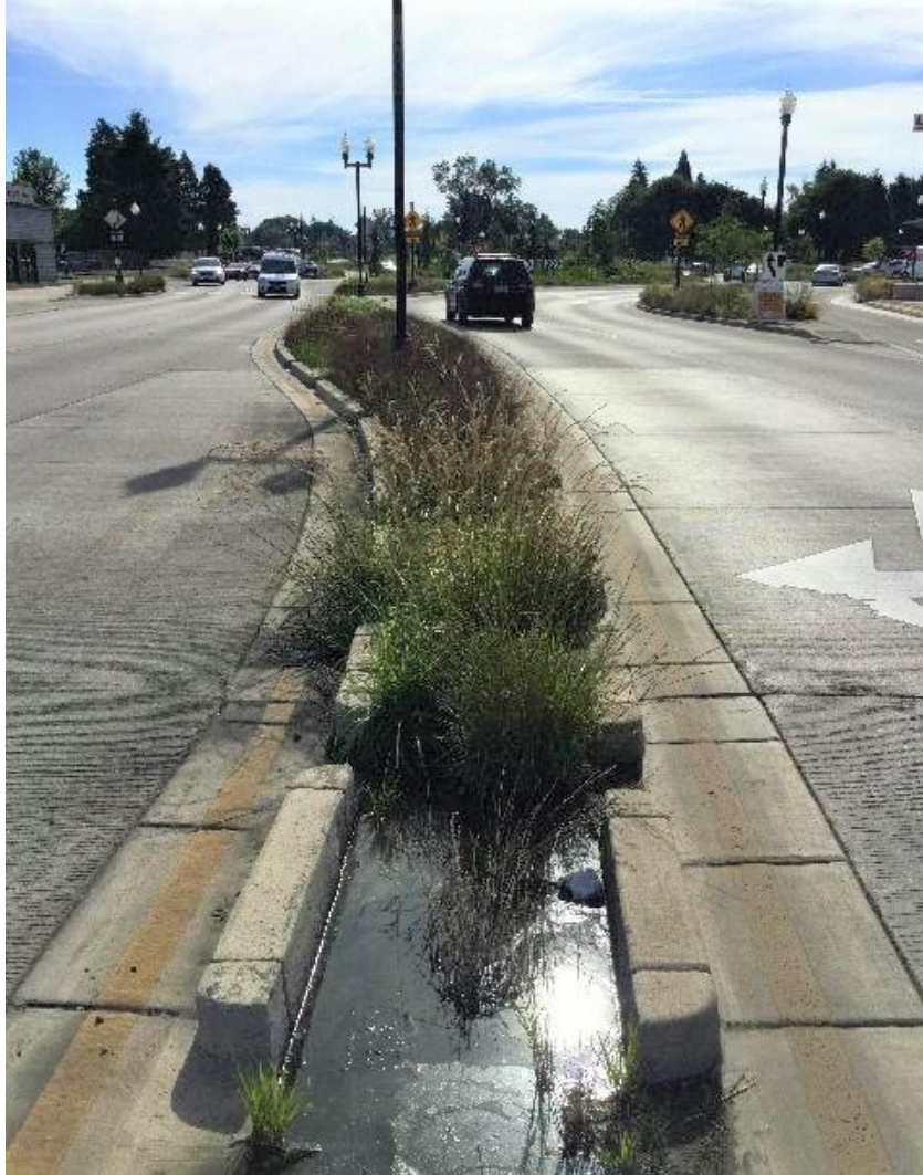
Franklin Blvd. Glenwood Planter 2021
