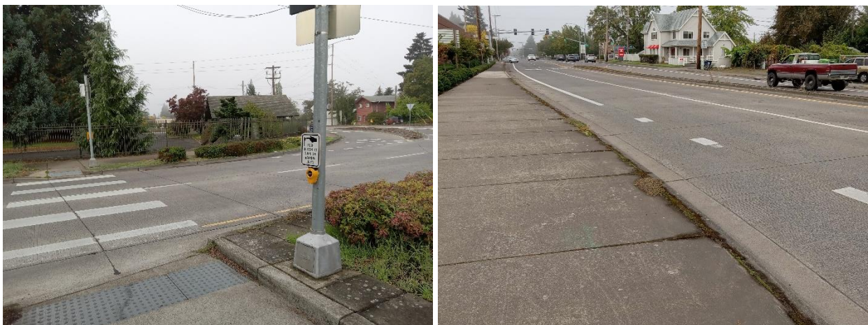
Pedestrian connections at the Harlow/Pioneer Parkway roundabout (right) and no curb ramp for people on bikes to exit the roadway before the roundabout (left).
