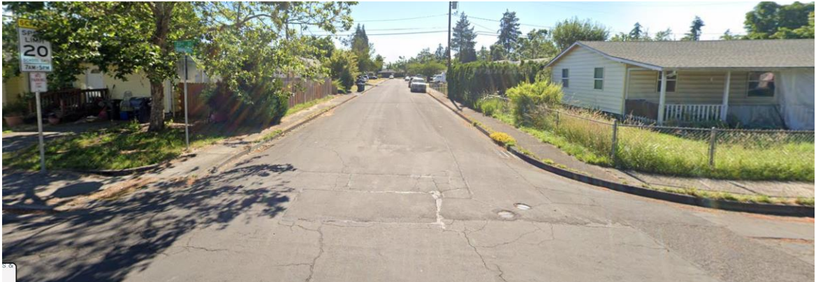
ADA curb ramps at Dubens and 23 rd St.
