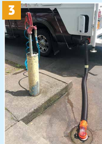
3 Bring your own sewer hose, connect it to the outlet, and drain your tank.
