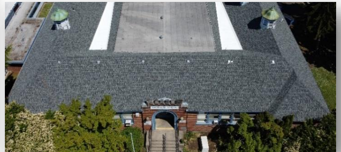
Whiteaker Head Start Community Center, highlighting the roof replacement
