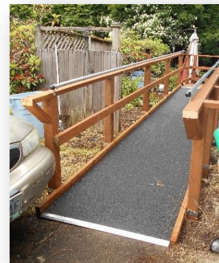
Access ramp, Eugene
