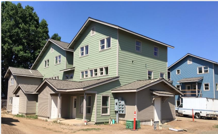
Iris Place under construction, Eugene
