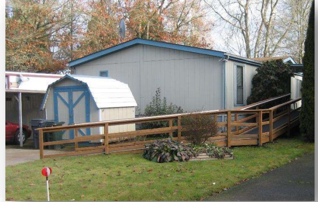
Wheelchair accessible ramp installed using CDBG funds, Eugene
