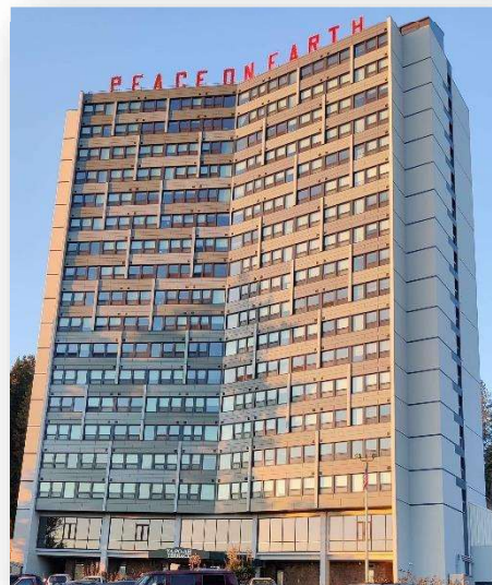
Ya-Po-Ah Terrace progress, Eugene
