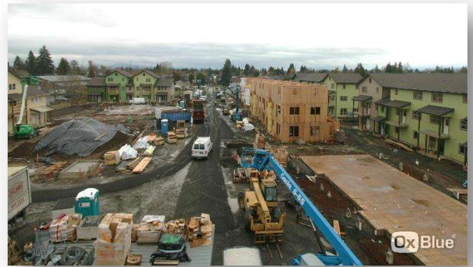
Sarang (formerly called Taney Place), under construction, Eugene
