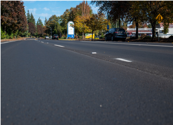
Centennial Blvd After
