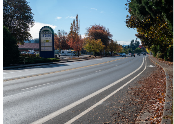
Centennial Blvd After
