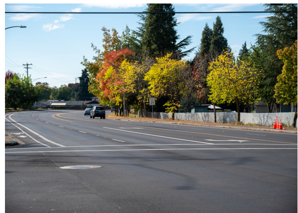
Centennial Blvd After
