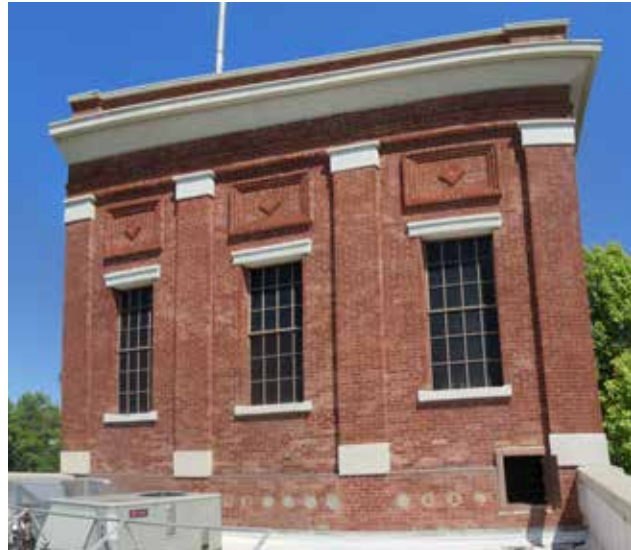
Figure 1-5: South elevation of 2nd story space from roof
