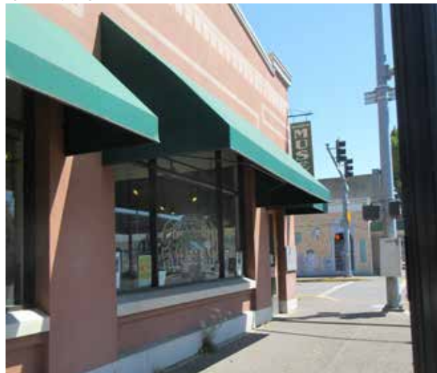
Figure 1-7: Main entry elevation
