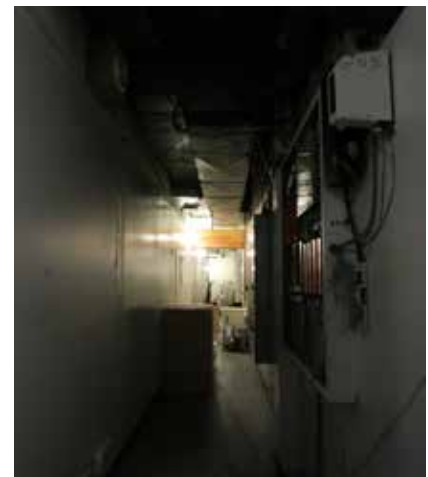
Figure 1-16: Booth Kelly blocked exist pathway
