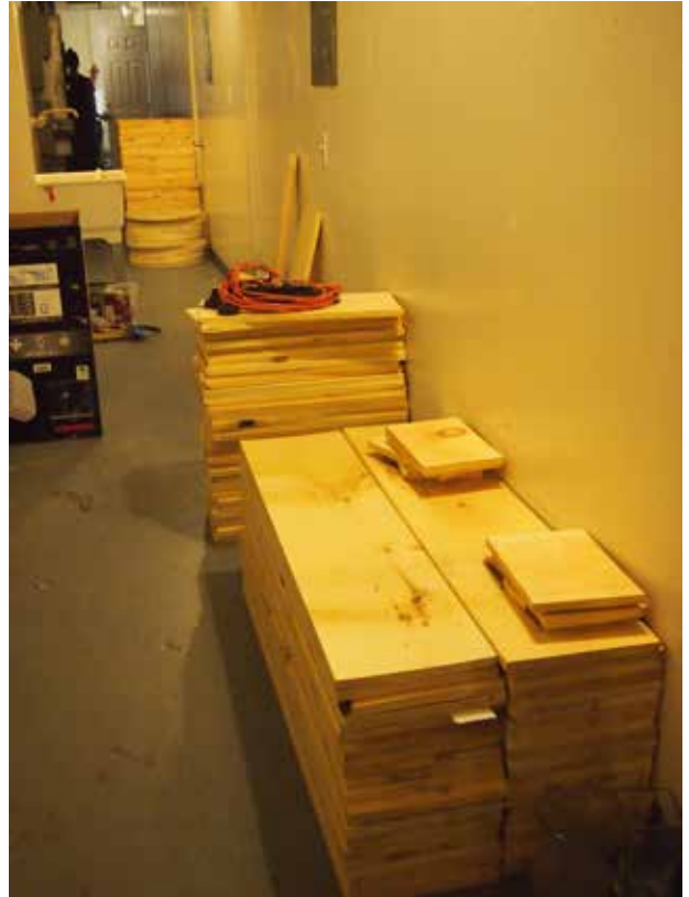
▲ Figure 1: The rear corridor of the Booth-Kelly off-site storage facility showing its use for storing flammable materials and generally being obstructed making safe and easy egress impossible. Specific space issues, as they impact the collections, will be discussed elsewhere in this document in the section headed "STORAGE".
