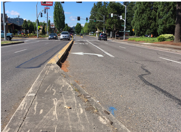
Mohawk Blvd Before
