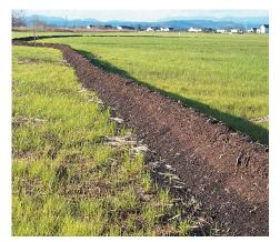
Compost berms are easy to install and they help keep construction pollution out of the stormwater system, and out of the river.
